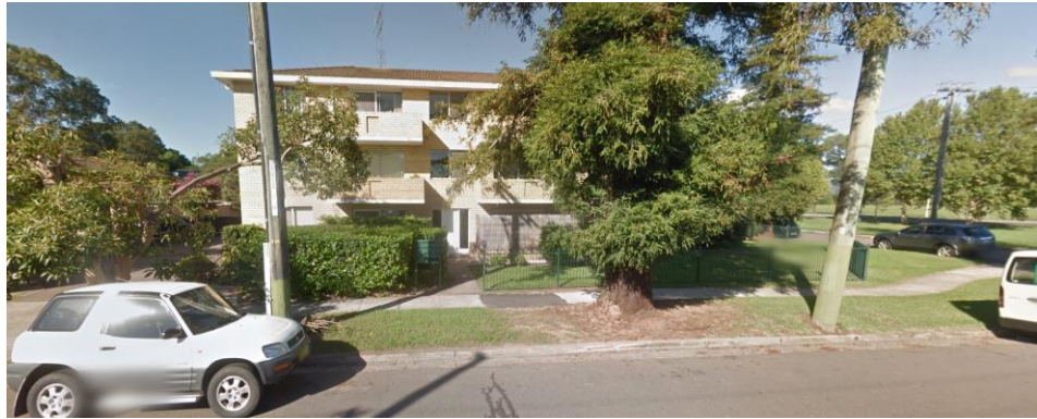
Figure 23 – Northern façade of 86 Union Road
